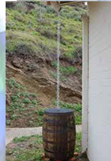
Rain Barrel using a Chain
