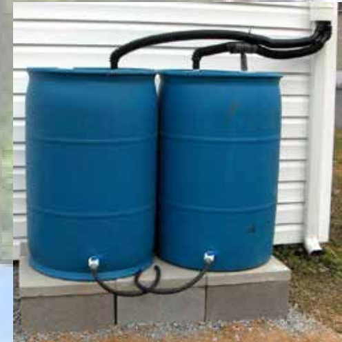
Multiple barrels can be connected together for increased storage.
